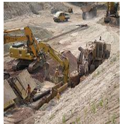
Slope instability issues for a temporary flood control levee in North Dakota, 2009
