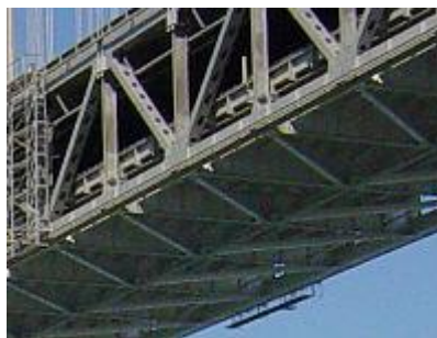
Additional diagonals were inserted under both decks of this bridge
