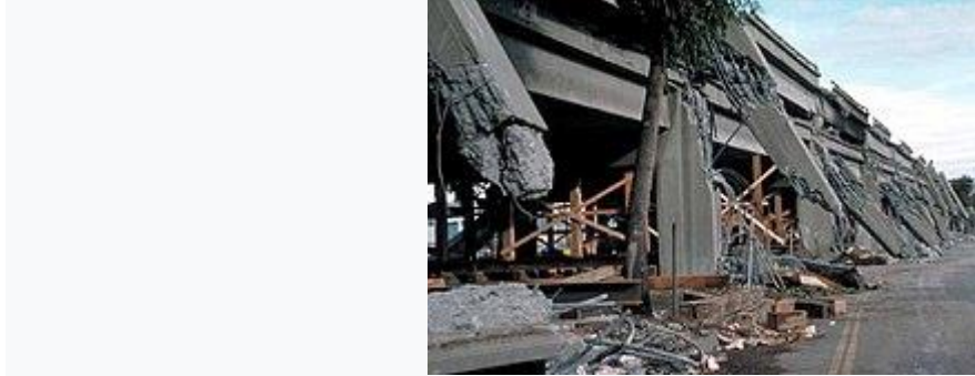
Cypress Freeway viaduct collapse. Note failure of inadequate anti-burst wrapping and lack of connection between upper and lower vertical elements.
