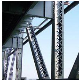
Obsolete riveted lattice members
