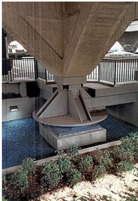
Close-up of abutment of seismically retrofitted Municipal Services Building in Glendale, California
