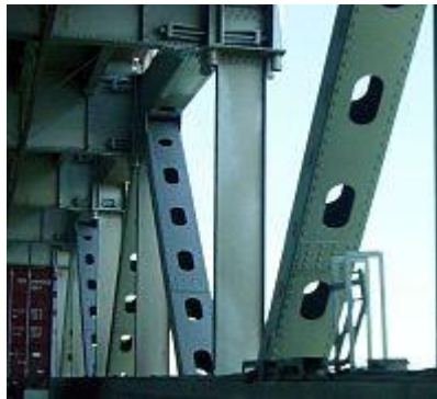
Bolted plate lattice replacement, forming box members
